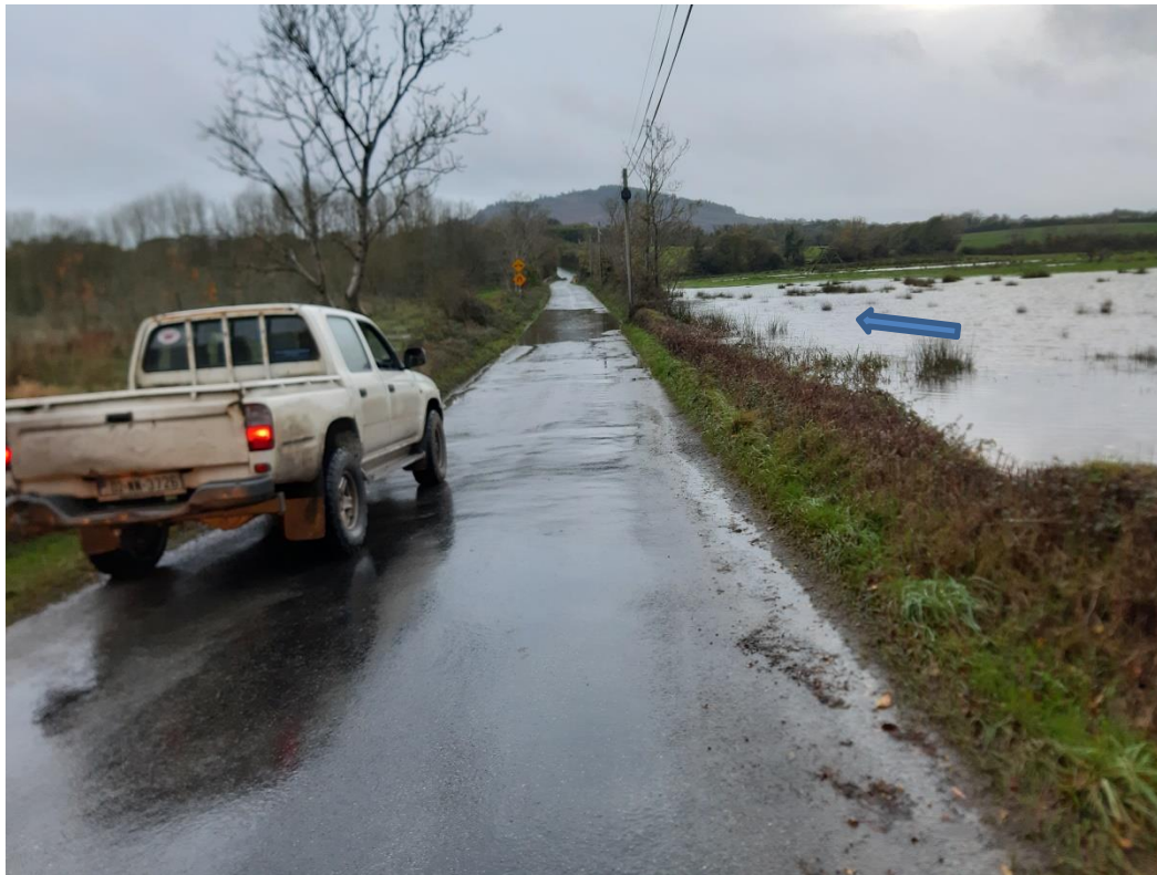
Fig.3 Inch River at Ahare Bridge in flooding conditions; road acting as a dam; looking south
